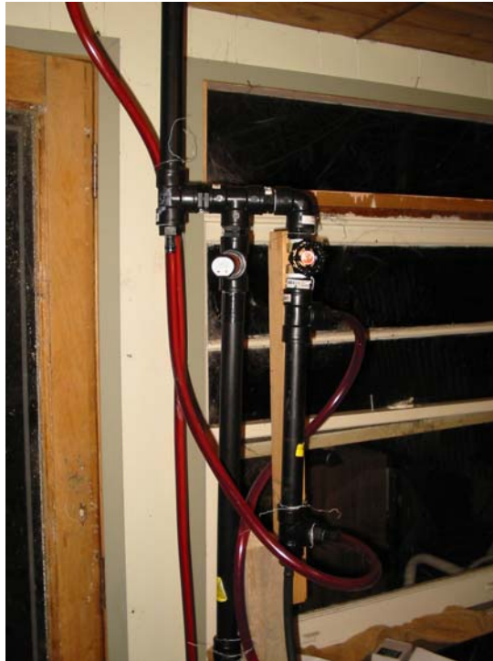
Figure 3 - Vapour management head
