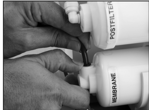
Fig. 20. Disconnecting Tubing from the RO Membrane
